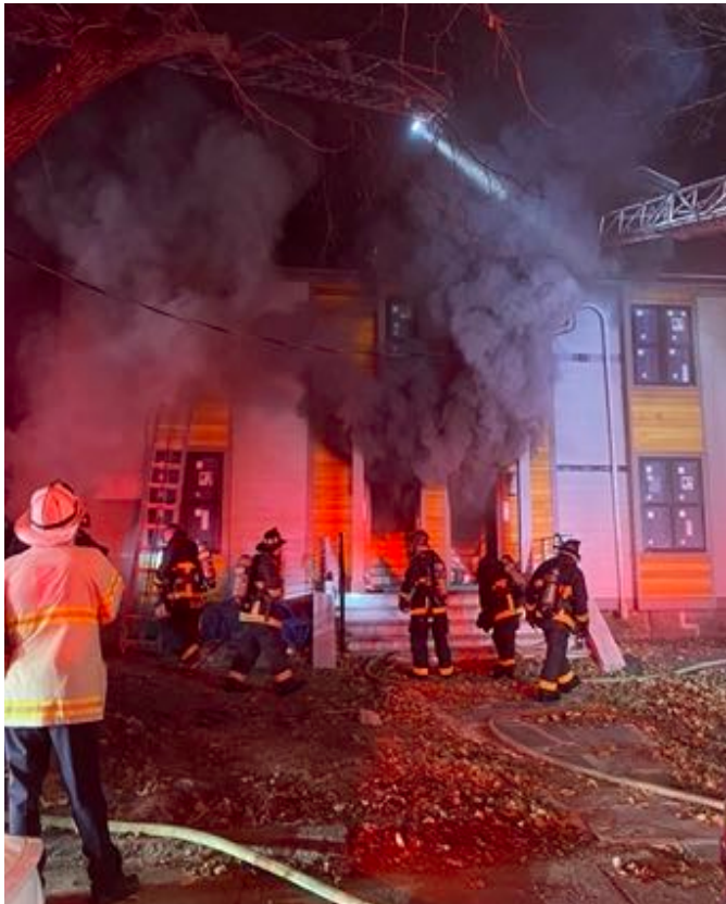
Below: Heavy caca chugging out of a building under construction at 1063 Washington St. Companies were ordered out and a second alarm transmitted for Box: 2-3478.
