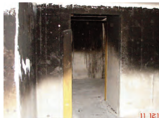
Figure C-7: Interior View of Burn Prop
