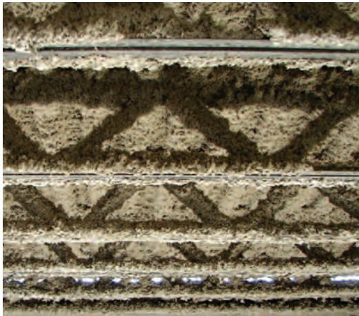
Figure C-4: Fireproofing added to structural steel
