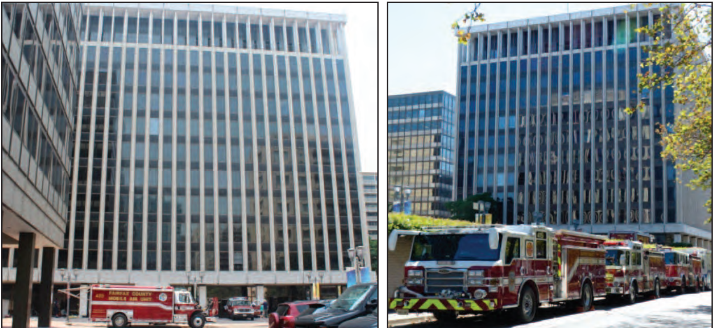
Figure 1: High-rise building located at 223 23rd Street, Crystal City, VA
