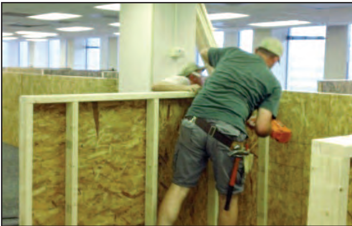
Figure 2: Office cubicle props on fire floor (10th)
