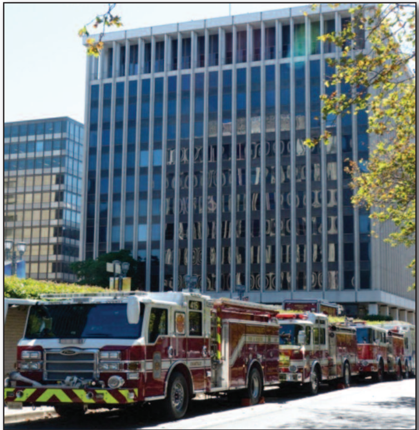
Vacant high-rise office building used to conduct field experiments in Crystal City, Virginia.
