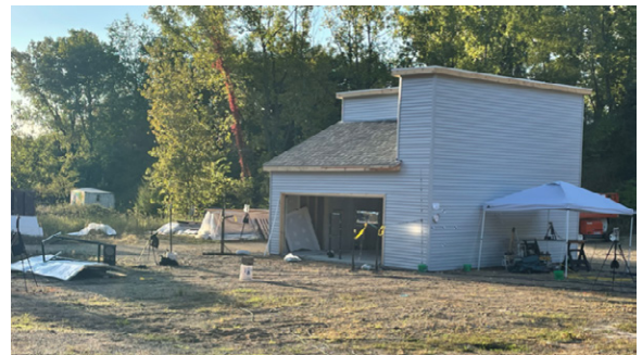
Notice the location of the door after the deflagration.
