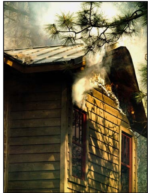
Figure 4.13. Firefighters must evaluate ember traps such as gable end and foundation vents, where embers can enter and ignite a structure. Photo courtesy of Kari Greer.
